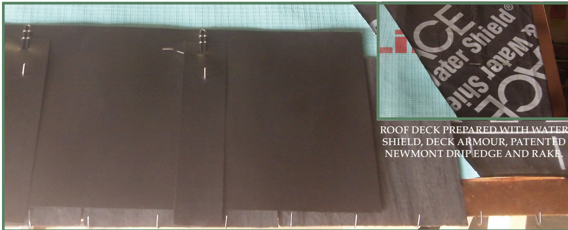
PREPARED ROOF DECK WITH STARTER / UNDER EVE SLATES BENEATH FIRST SLATE SHIELD PANEL IN DRIP EDGE.
