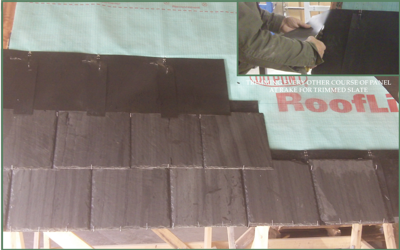
THIRD COURSE SLATE SHIELD™ SLATES BEING INSTALLED- PLEASE NOTE TRIMMED PANEL AT RAKE.
