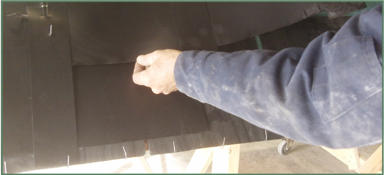
SLATE SHIELD™ PANEL IN DRIP EDGE WITH NEXT PANEL BEING INSTALLED – PLEASE NOTE . PANEL IS INSERTED/TUCKED BENEATH THE LAST EXTENDER STRIP OF THE PREVIOUS SLATE SHIELD™ PANEL
