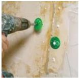
Use the plastic washers and screws to clamp the plaster into "soft contact" with the lath—pulling the plaster to just touch the lath, while leaving room for the adhesive to flex. In 24 hours, after the adhesive has cured, remove the clamps. The plaster is now stable, bridged subsurface with the lath, and will not re-crack.
