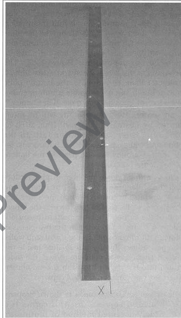
Figure 1-33. Bottom plate shot down following the wall line with the plate sitting on the side of the wall line marked with an X.
