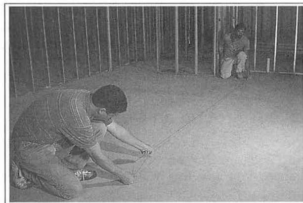
Figure 1-16. Here the chalk line has been set and is ready to snap.
