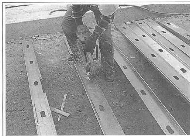
Figure 1-73. Cutting down the hard side of a structural stud using a Quickie Saw.
