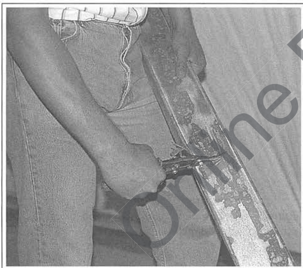
Figure 1-68. Cutting into the hard side of the stud, beginning at the bottom notch mark.
