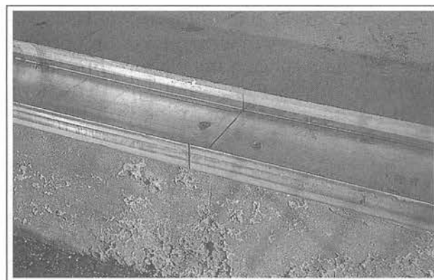
Figure 1-34. Bottom plate on a 6-inch structural stud wall butted together and shot down.
