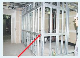
Additional hollow section for bracing and load bearing steel stud
